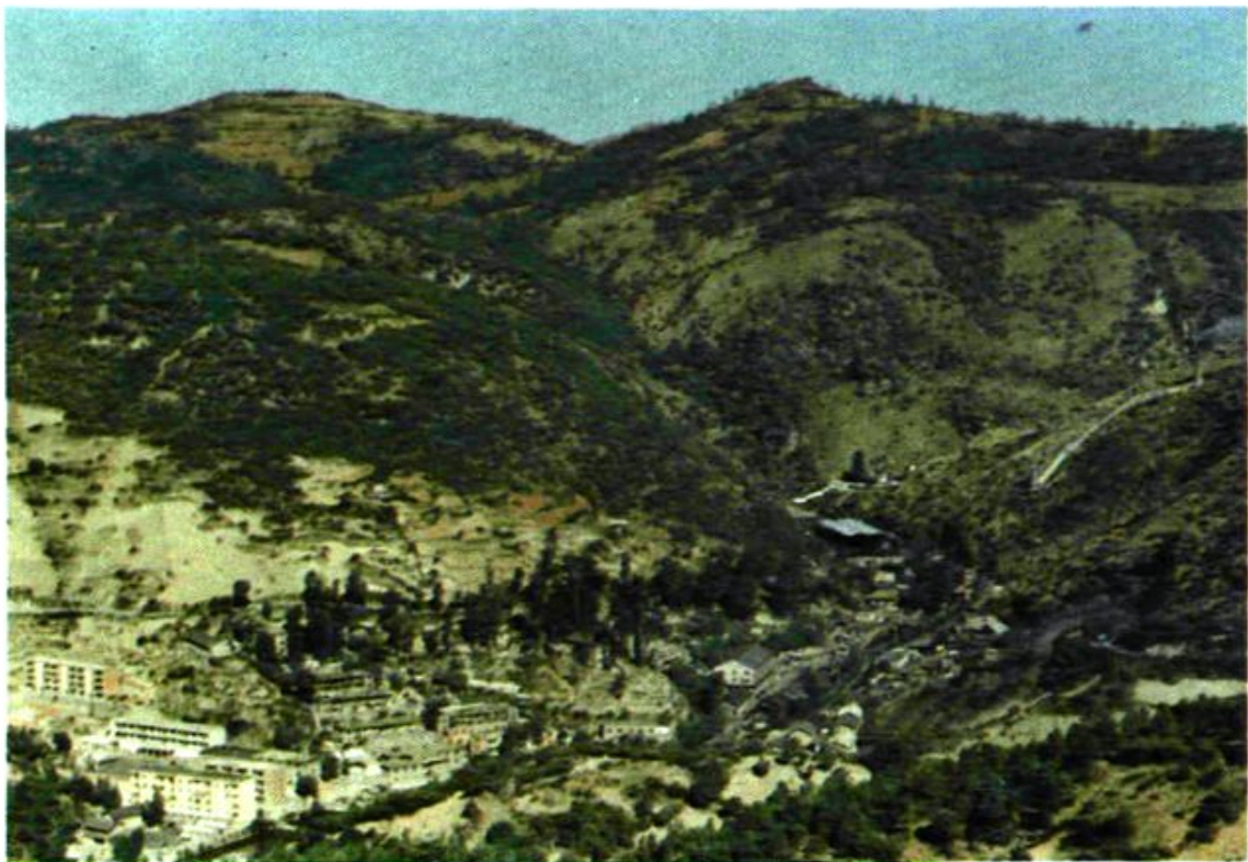
喷水洞电厂全貌
