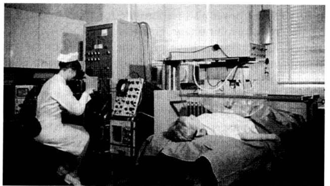
Figure 1-2 Dr. Lehman used a water path system to scan his obstetric patients.
