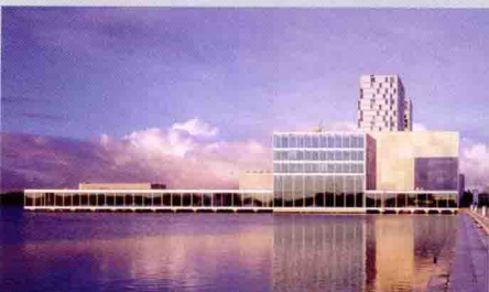
'De Kunstlinie' Theater and Cultural Center, Almere 阿尔梅勒“艺术线”剧院与文化中心 Theater, culture center, restaurant, café Almere, The Netherlands 1998.02-2004.08 2004.09-2006.10 2006.10
