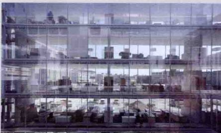
Novartis Campus WSJ-158 诺华园WSJ-158 Office Basel, Switzerland 2003.12-2005.03 2005.03-2006.09 2006.09
