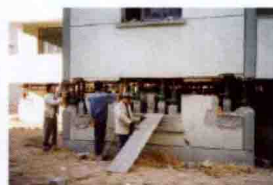
“轮番顶升法”顶升八层楼房
