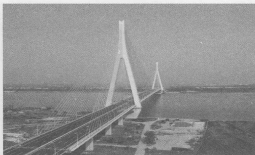
b) 斜拉桥—跨过江，江中无墩——鄂东长江大桥 Stayed-cable bridge—Erdong Yangtze bridge
