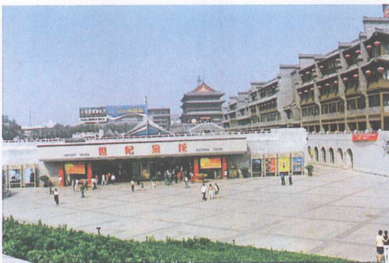
彩图 7-31(b) 西安钟鼓楼广场地下商场出入口 C. P. 7-31(b) The entrance of xian Bell-Drum Tower square's underground shopping center
