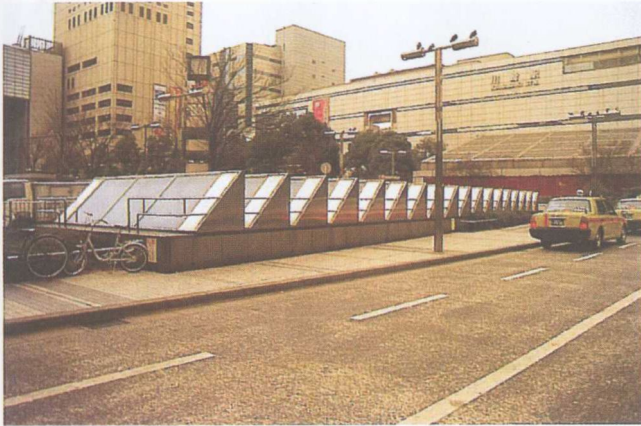
彩图 7-10(b) 图 7-10(a)的地下街锯齿天窗采光景观 C. P. 7-10(b) The skylight of C. P. 7-10(a)'s "Chigakai"
