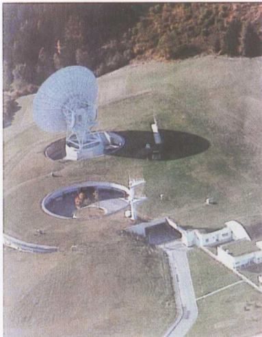
彩图 7-9 澳大利亚某掩土建筑卫星中继站 C. P. 7-9 The earth sheltered building of a satellite relay station, Australia
