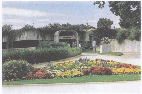
彩图 7-4(a) 法国某市政府地下建筑出入口 C. P. 7-4(a) The entrance of a city government's underground building, France
