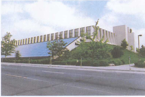
彩图 7-5(d) 前述太阳房向阳面太阳能集热器 C. P. 7-5(d) The large area solar collector on the sunfacing side of the control Data center, Minneapolis, USA
