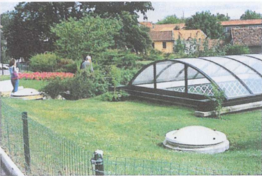
彩图 7-4(b) 法国某市政府地下建筑屋顶绿化及下沉式温室 C. P. 7-4(b) The roof greening and sunken greenhouse of a city government's underground building, France
