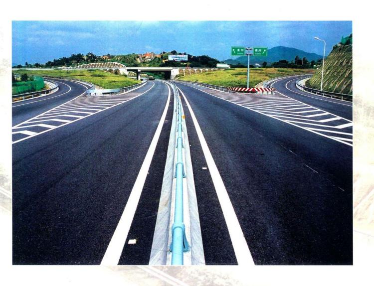
The expressway is 154 kilometers long starting from Yingqian, Changle City in the north and ending at Xifu, Quanzhou City in the south. A-11.49-kilometer-long road connects Yingqian with Fuzhou. The width of the trunk roadbed is 26 meters. It is a two-way road with 4 driving lanes. The designed driving speed is 120 kilometers per hour. The whole line is equipped with corresponding service areas, toll stations and communication monitoring systems. The total investment is RMB 4.67 billion yuan.
