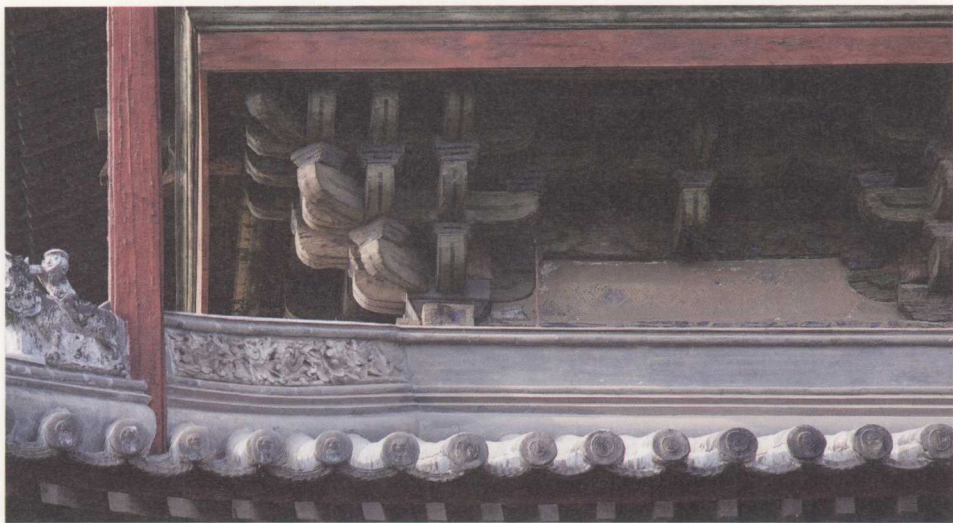
观音阁柱头及补间铺作斗拱
