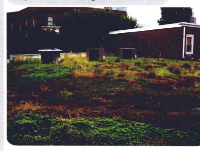
and temperature differences of, 35°C during the year and 15°C over 24 hours are not usually exceeded. In addition, the Green Roof creates a protection layer for the waterproofing in case of mechanical damage like hail, wind, vandalism, and fireworks.
