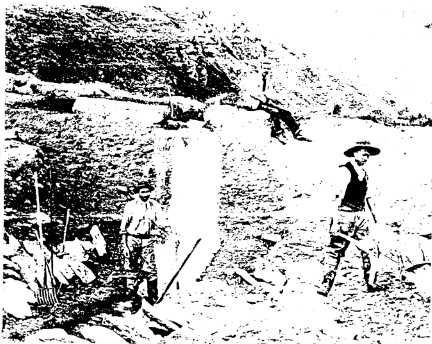
Removing the large rocks from a sluicing claim at Waiakata, Winding Creek. The wide (sluice) fork on the left was used for lifting the smaller rocks from the tailrace. Photograph from the Ing Collection. Alexander Turnbull Library.
