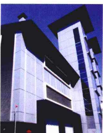
警察训练学校战术训练大楼 Tactical Training Complex at Police Training School
