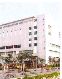
三家村市政大厦 Sam Ka Tsuen Municipal Services Building
