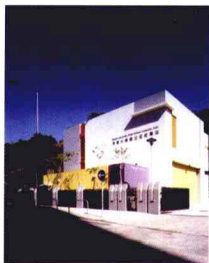
浸会大学道垃圾收集站及苗圃 RCP and Transit Nursery at Baptist University Road
