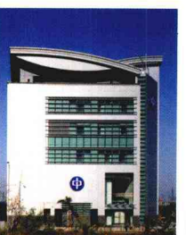
西九龙中华电力百周年变电站 CLP Power Centenary Substation at West Kowloon Reclamation "A"
