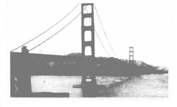
and, at the middle point, 70 metres above the water of San Francisco Bay. The main cables that hold the bridge are one metre in diameter. The bridge can safely withstand winds of up to 160 kilometres an hour, and it can sway as much as 8 metres in strong winds.
