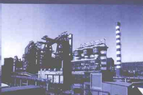
首钢为津巴布韦钢厂建造的1600立方米高炉是迄今为 止该国最大的高炉 The 1600 cubic meters furnace built by Capital Steel for Jin Ba Biwei Steel Factory is the largest blast furnace up to now
