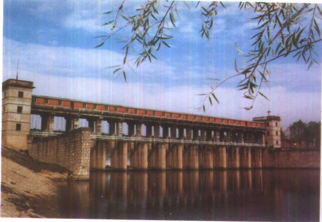
临泉县杨桥分洪闸
