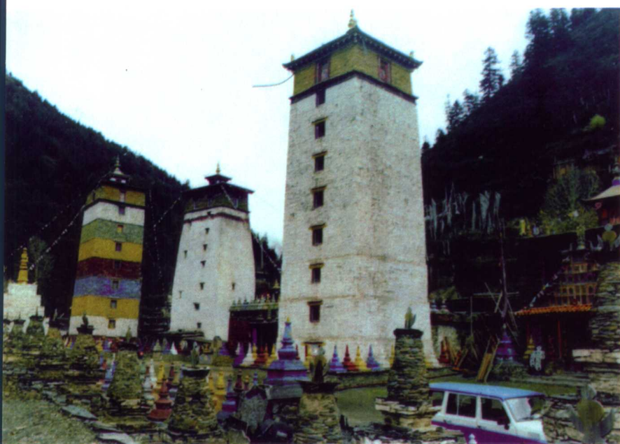
壤塘觉囊寺转经楼 Prayer buildings of Jonang Monastery, Litang county.
