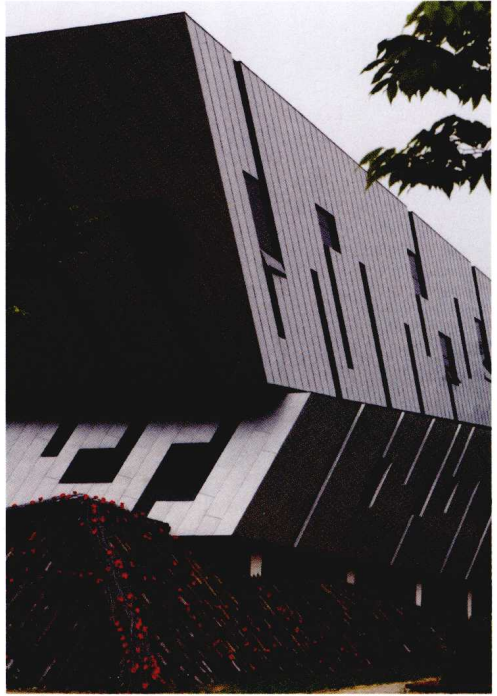
The geometric windows were designed after the shape of a PCV electric circuit.
