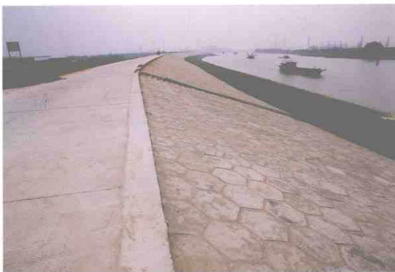
▲固若金汤的南海市堤坝
