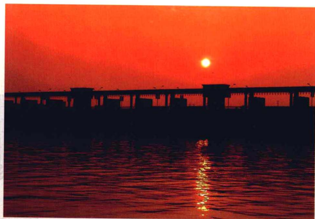
潇湘水电站大坝
