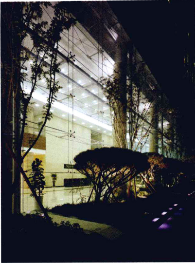
Night view of the lower exterior
