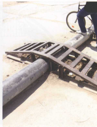
Uninsulated district heating pipeline in a residential area.
