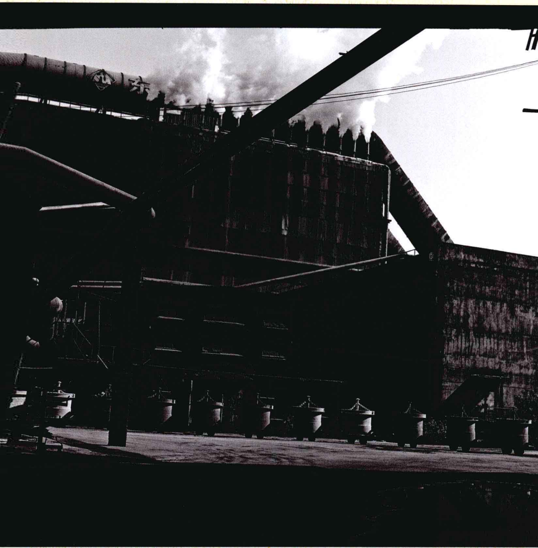
宝钢集团上钢三厂 The Third Branch of Shanghai Bao Steel Corporation, 2002
