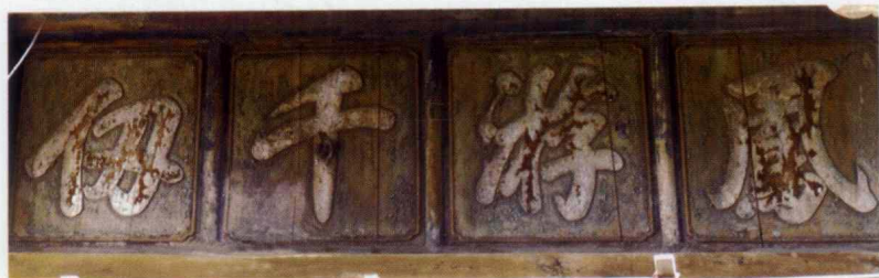
正厅东一间门池“凤游千仞”字样
