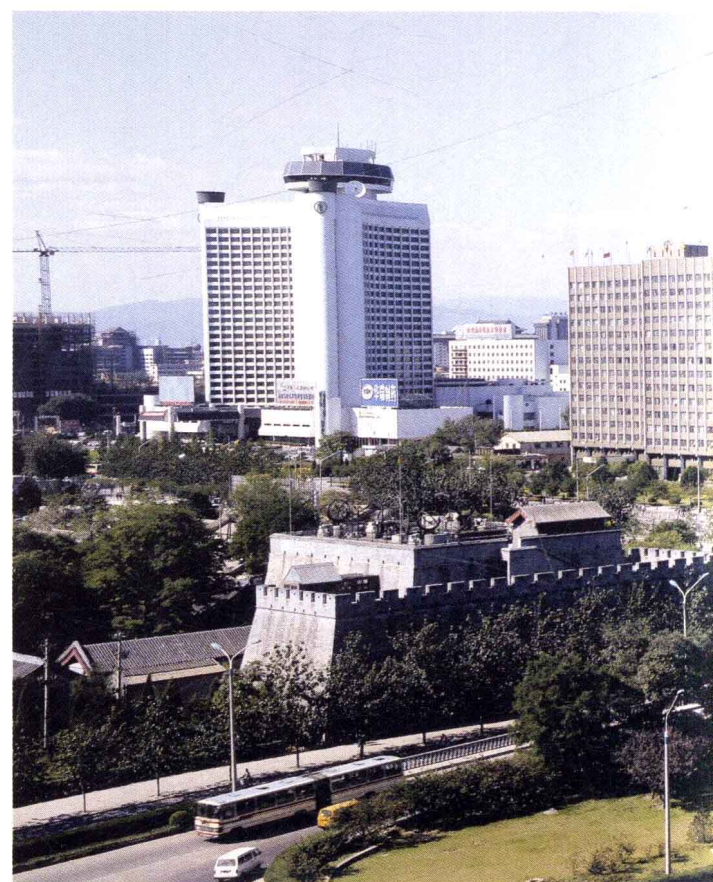
建国门立交桥 The Jianguomen Flyover
