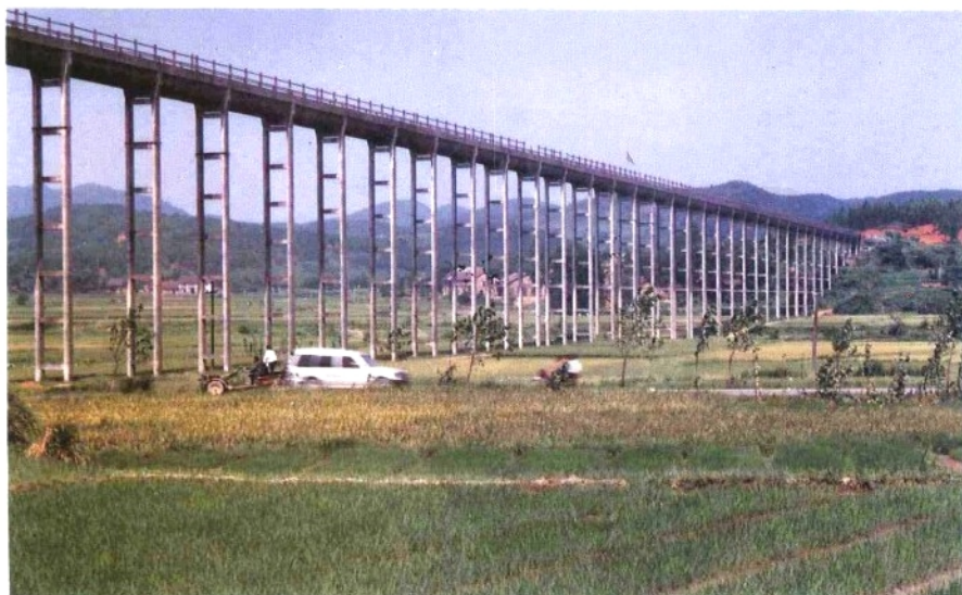
龙海乡茨冲渡槽
