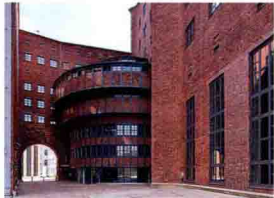
17. Electrical Substation at Buchhändlerhof Hans Heinrich Müller (p. 53)
