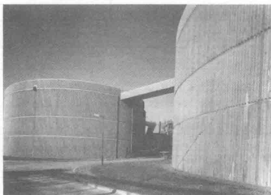
Fig. 1-11 Circular concrete tanks used as a part of the wastewater purification facility at Howden, England (Northumbrian Water Authority with Luder and Jones, Architects).
