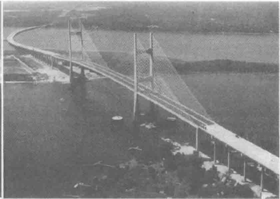
Fig. 1-8 Napoleon Bonaparte Broward Bridge, with a 1300 ft center span at Dame Point, Jacksonville, Florida (HNTB Corporation, Kansas City, Missouri).
