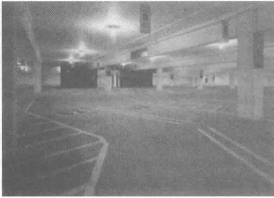
Fig. 1-1 One-way reinforced concrete floor slab with monolithic supporting beams (Portland Cement Association).
