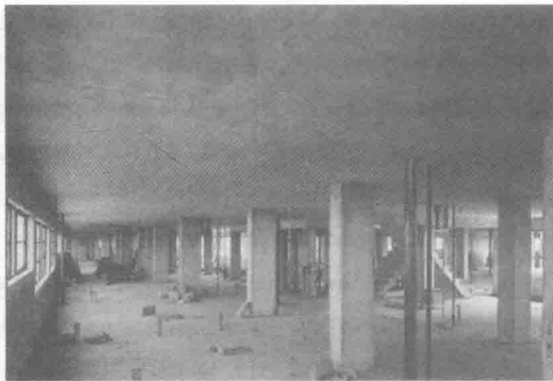
Fig. 1-3 Flat plate floor slab, carried directly by columns without beams or girders (Portland Cement Association).
