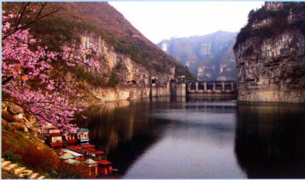
观音岩水电厂水库大坝
