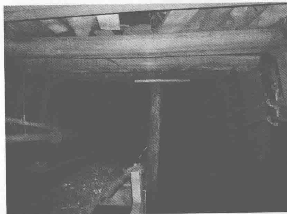
图7 运煤巷道底鼓边帮顶板严重挤压破坏(被迫停产处理)
