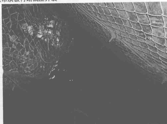
图7 运煤巷道底鼓边帮顶板严重挤压破坏(被迫停产处理)
