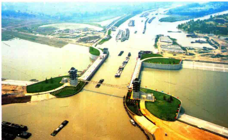
The China Grand Canal, inscribed on the UNESCO World Heritage List in 2014. A waterway “flyover” at the junction of the China Grand Canal and the North Jiangsu Main Irrigation Canal, Huai'an, Jiangsu Province, China.
