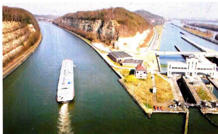
Lock Lanaye, Albert Canal, Belgium.
