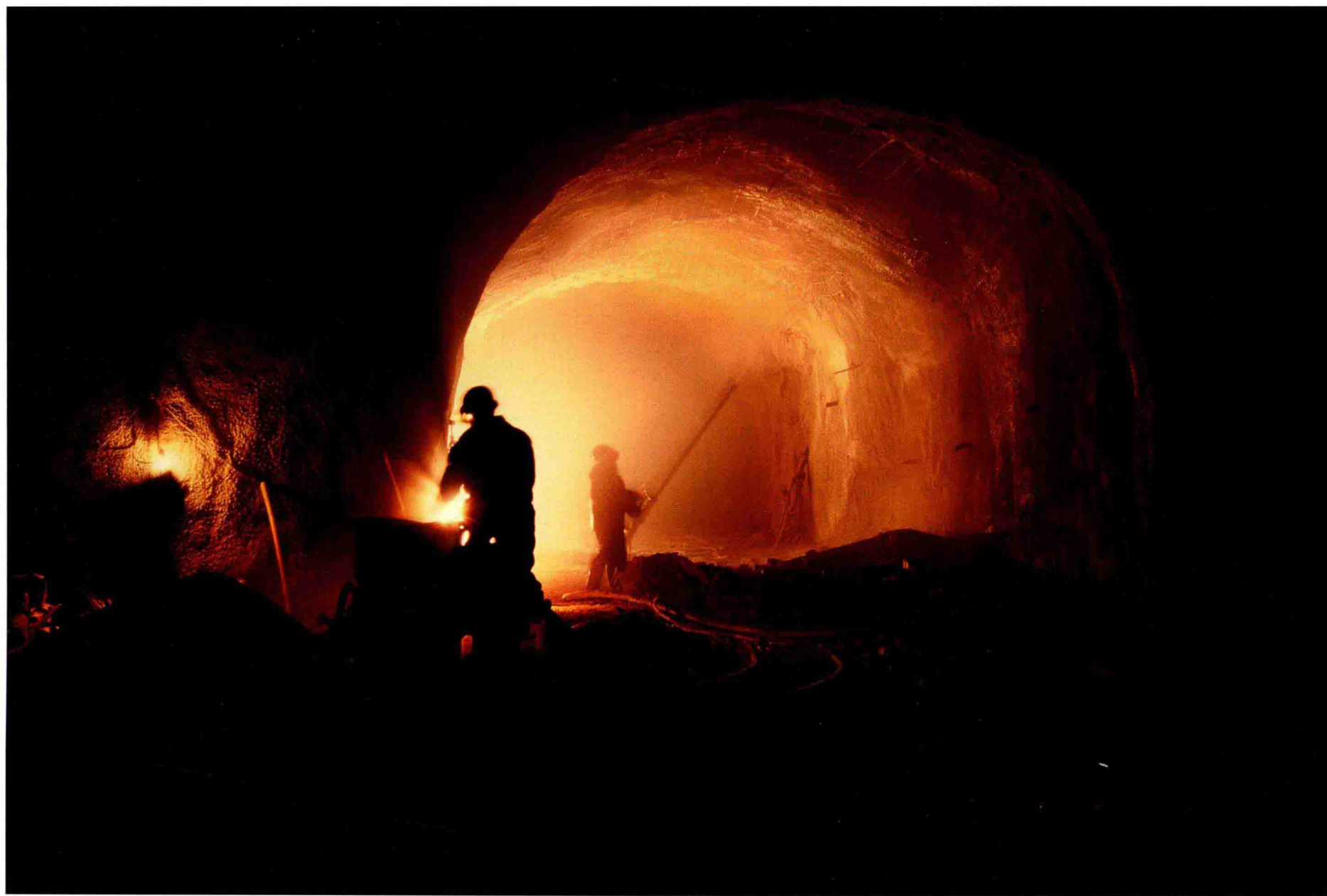
● 锚杆支架喷浆 ●
