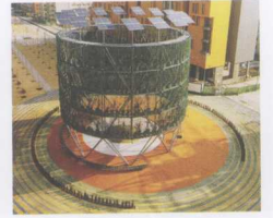
30. Vallecas Ecoboulevard, Madrid outskirts Ecosistema Urbano architects Ltd. Madrid, Spain, 2007
