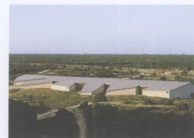
5. Centre for Visitors of the Marineworld Cruz y Ortiz Arquitectos Huelva, Spain, 2001
