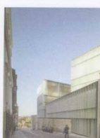
98. Rehabilitation and Expansion of the Eamos Carrion Theatre MGM Arquitectos Zamora, Spain, 2013
