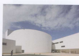
69. Manzana del Revellín Cultural Center Álvaro Siza Vieira Ceuta, Spain, 2010
