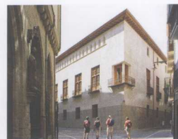
44. Constable's House Tabuenca & Leache Arquitectos Navarra, Spain, 2008
