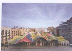
17. Rehabilitation of Santa Caterina Market Enric Miralles + Benedetta Tagliabue Barcelona, Spain, 2005 (p. 124)
