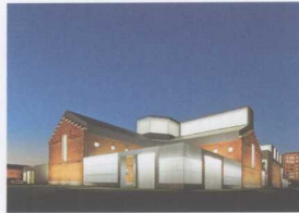
83. Rehabilitation of Former Prison of Palencia as Cultural Civic Center Exit Architects Palencia, Spain, 2011
