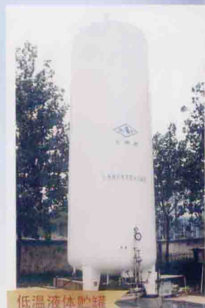
低温液体贮罐
