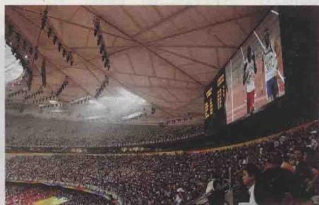
No matter where you are seated, the distance to the central point of the arena is about 140 meters. The excellent acoustic design ensures that everyone inside can clearly hear what is going on. In every detail the design is optimized to guarantee the best ventilation and maximum use of natural light, even when the stadium is full.
