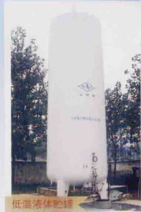
低温液体贮罐
