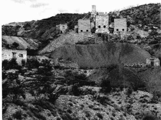
Figure 3 Three eras of mining activity on Mariscal Mountain are visible in this view. At the lower right are the Ellis era ruins; in the middle are the Mariscal era ruins; and at the upper left are the Viviana era ruins. The mine entrance is at the top left. The piles of tailings (waste rock from the furnace) are prominent directly below the ruins of their associated era. Photo by Bruce Harms.
