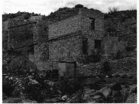
Figure 5 The top floor and the roof are missing in this interior view of the office structure. Firebricks were mixed with stone from the site to build the first floor, while firebrick alone was used to form slots for the floor joists (middle of image) and roof joists (top). Photo by Bruce Harms.
