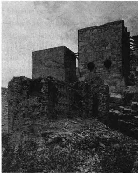
Figure 1 The ruins of the Mariscal Scott furnace (foreground) are only one-third the height of the complete furnace. Behind the furnace are two of the three mercury condensers. HAER photo by Bruce Harms.
