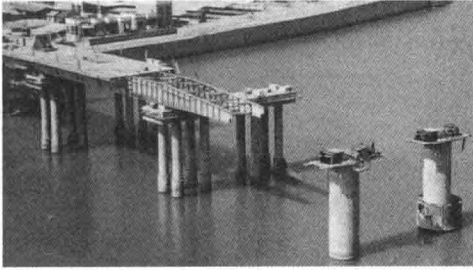
图 1-6 顶推施工
