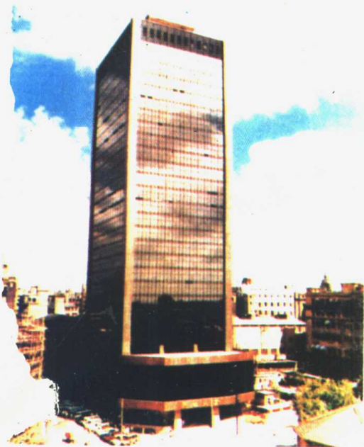
The Union Building, Shanghai 上海聯誼大廈
