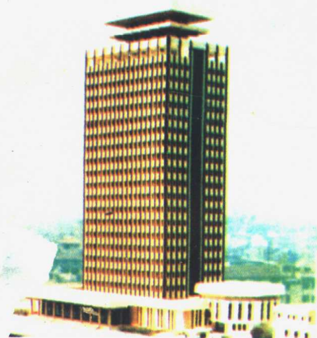
Telecommunication Building, Shanghai 上海電信大樓
