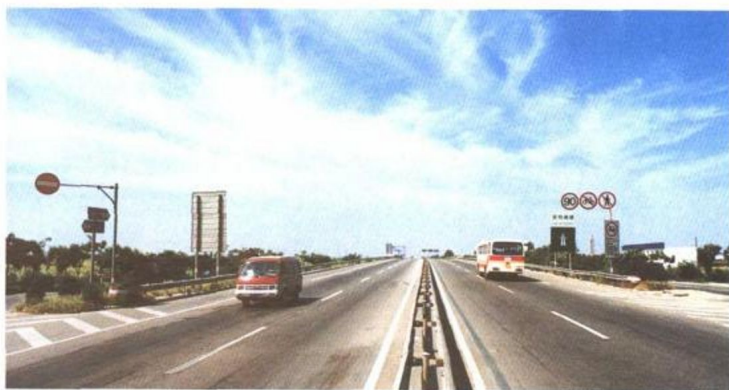
●京哈高速直通三河 Jing-Ha Highway directly run through Sanhe.
