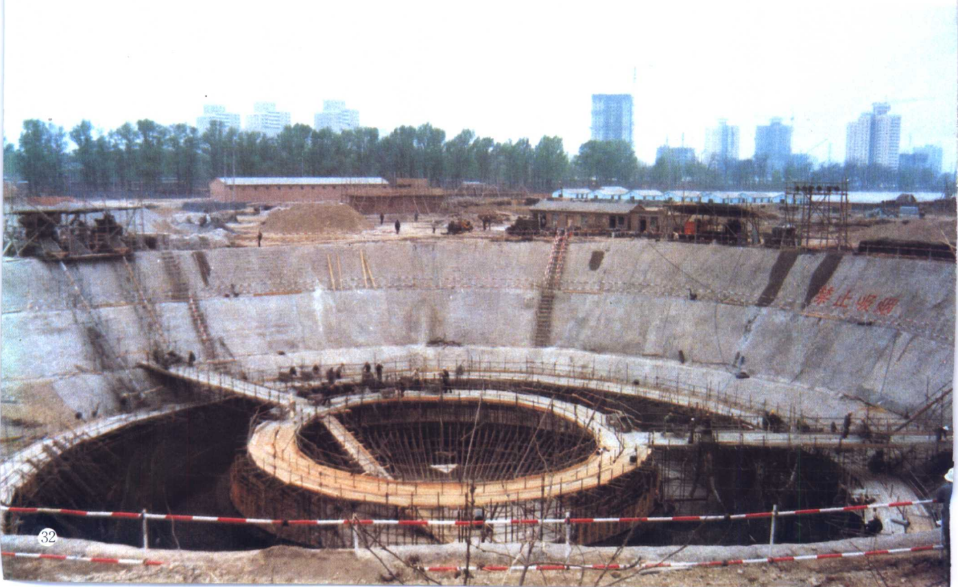
32 中央电视发射塔塔基施工 Base of Central TV Transmission Tower under construction
