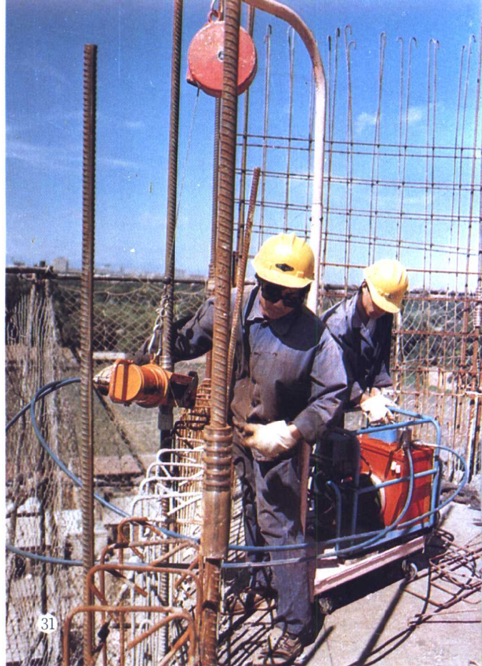
31 中央电视发射塔钢筋挤压连接 Extruded connection of reinforcing bars of Central TV Transmission Tower
