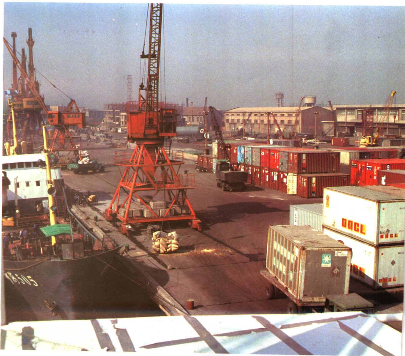
宁波港镇海港区 Ningbo Port: The Zhenhai harbour
