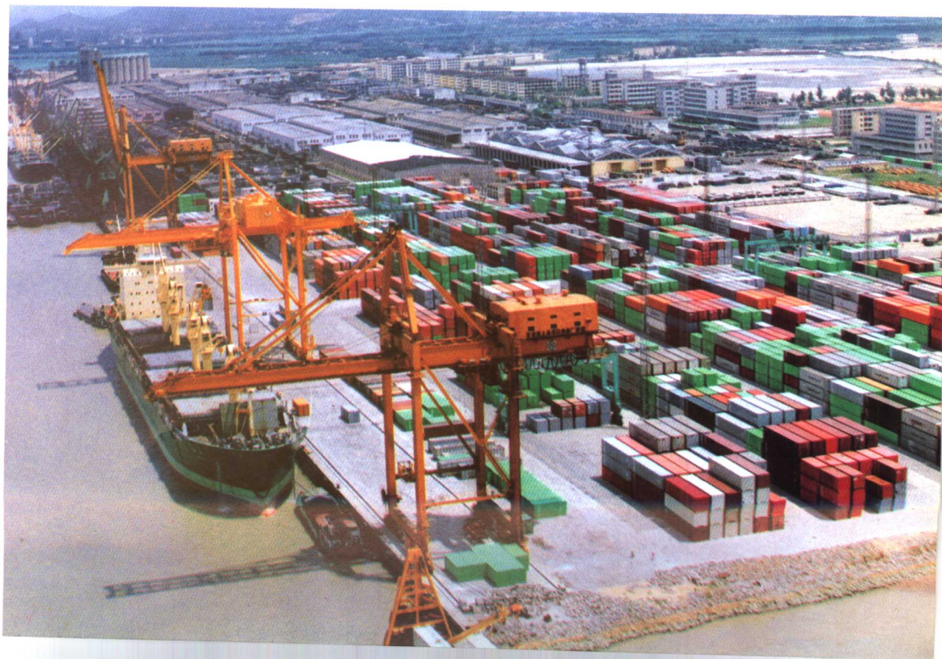
广州港黄埔港区集装箱码头 Guangzhou Port: The container terminal of Huangpu Harbour
