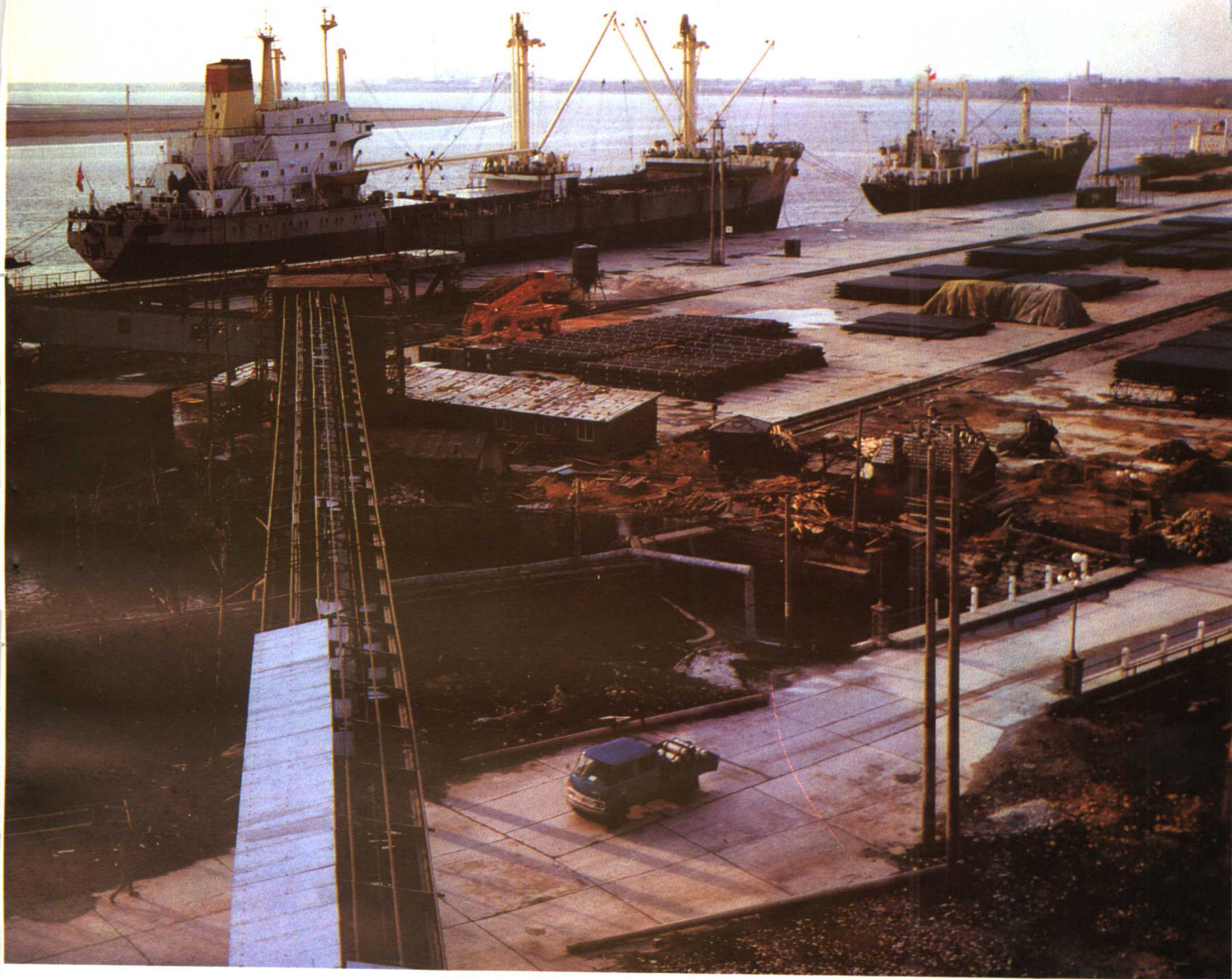
营口港鲅鱼圈煤码头 Yingkou Port: The Bayuquan coal wharf
