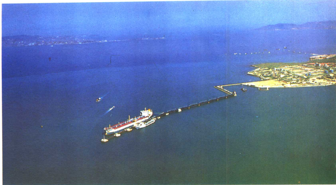
青岛港黄岛油码头 Qingdao Port: The Huangdao oil terminal
