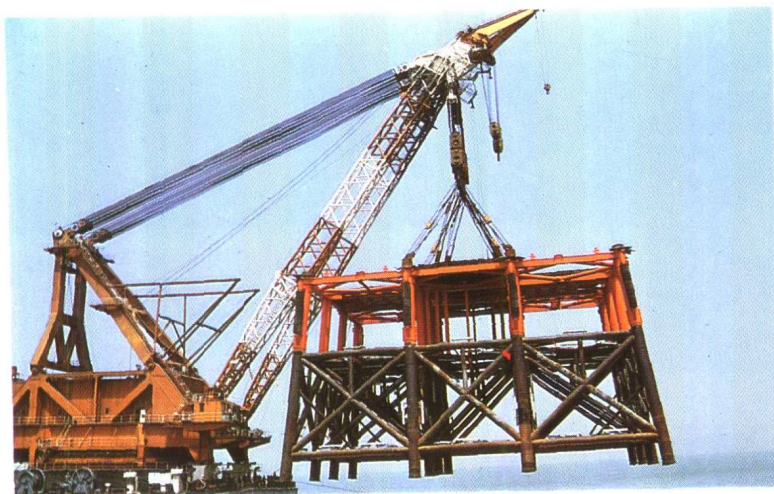
"DA LI HAO" floating crane with a lifting capacity of 2,500t. Photo shows her lifting China's first offshore jacket
