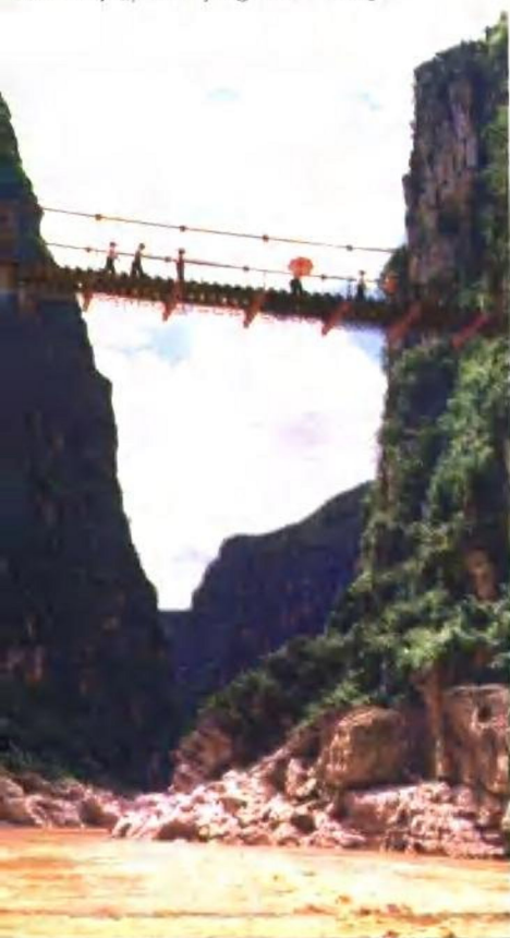
花江铁索桥 Hua jiang chain bridge
