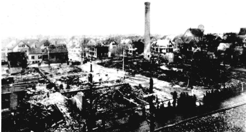
Figure 1.2 Shoe factory after the boiler explosion of March 20, 1905, which led to the adoption of many state boiler codes and the ASME Boiler and Pressure Vessel Code . (Courtesy of The Hartford Steam Boiler Inspection and Insurance Company .)
