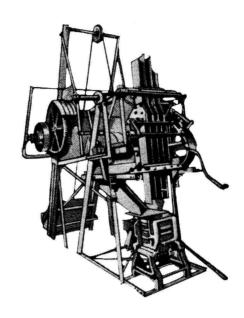
CONCRETE block-making machine, circa 1909.
