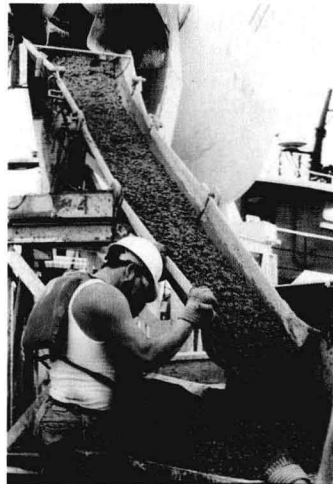
Fig. 1-5. Workable concrete should flow sluggishly into place without segregation. (59292)
