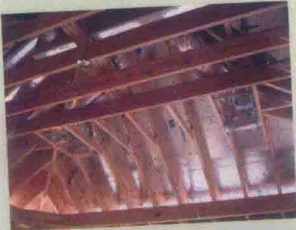
Figure 2.13a Radiant barriers may be applied in the factory to the roof decking for easy installation. LP's TechShield is OSB with a perforated radiant barrier that reduces radiant heat transfer and allows moisture drying.
