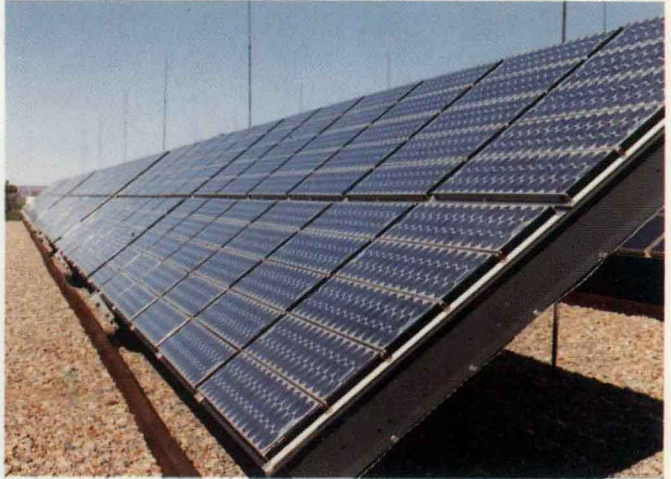
(11) A 100kW monocrystal Si solar cell array (Natural Bridges National Monument, Utah).
