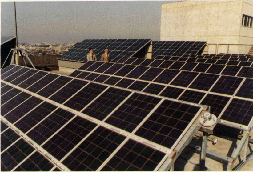
(7) A 2.5kW power generation system employing amorphous Si solar cells (at O-okayama campus, Tokyo Institute of Technology).
