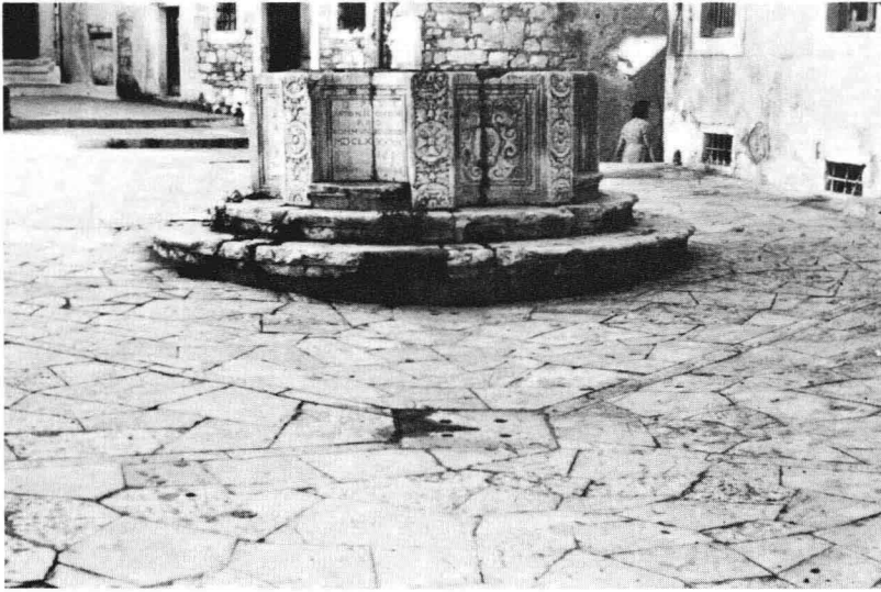
FIG. 1-1. Venetian cistern head located at Dubrovnik, Yugoslavia, showing a stone grating.
