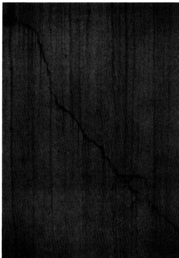
Fig. 1 a : The staircase leading to the lecture room on which the 1st Bolomey workshop took place shows a crack which is due to differential settlement.
