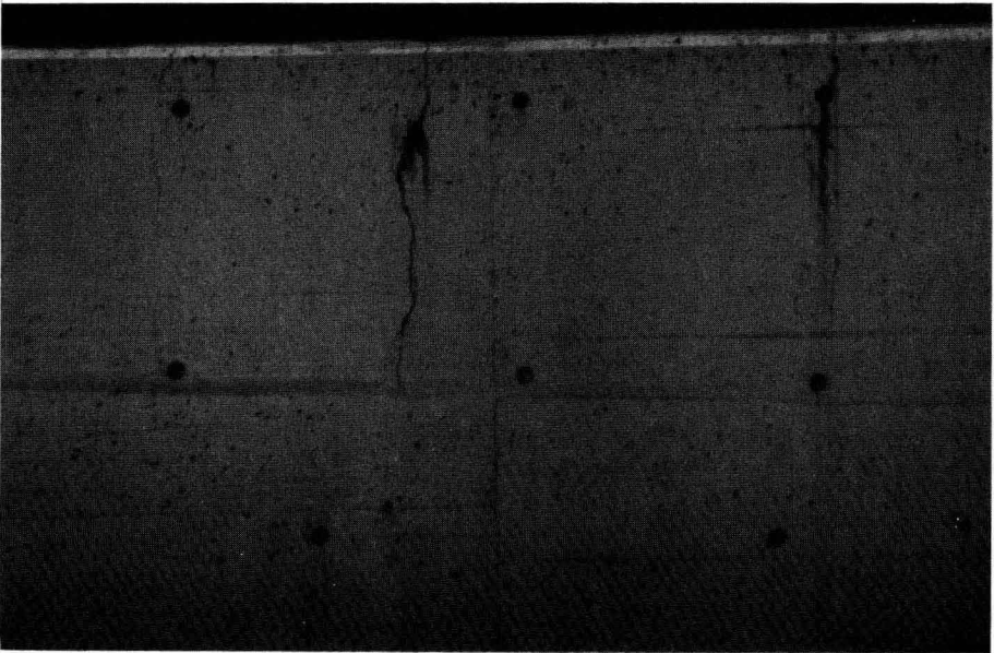
Fig. 1 b : A sustaining wall shows vertical cracks; the upper half is exposed on both sides to environmental conditions (drying and temperature variations)
