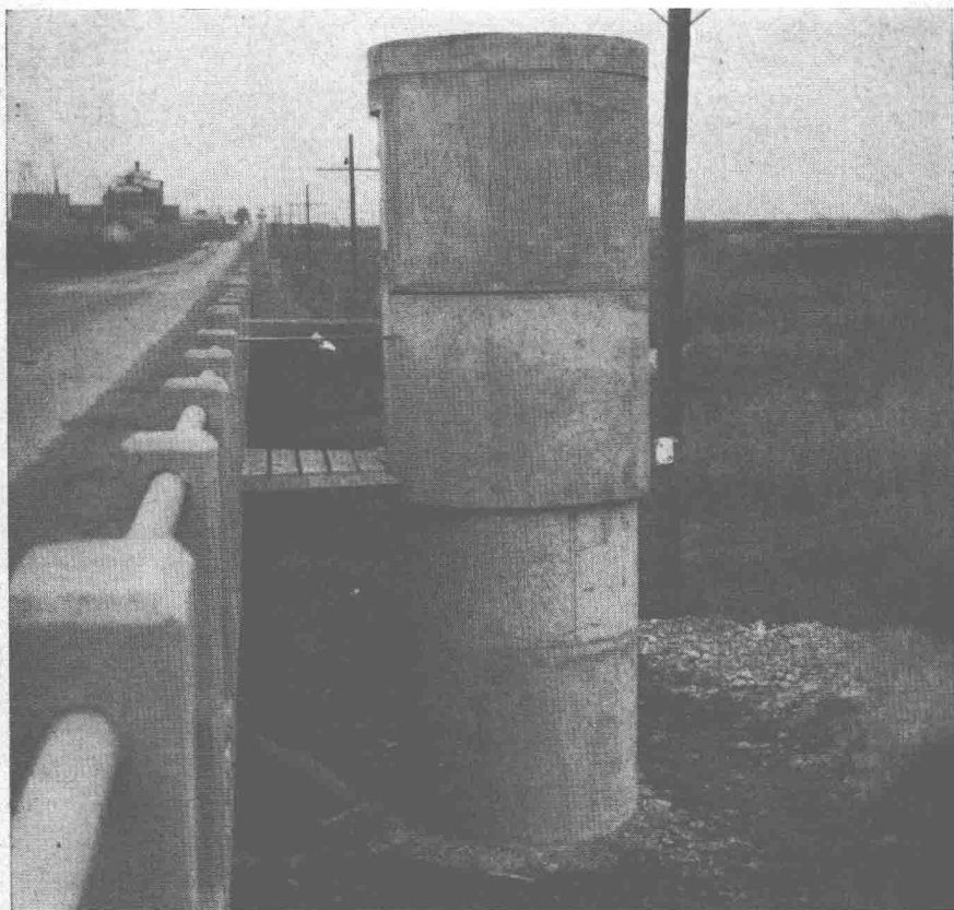
This unusual use of concrete pipe is a river gage house at Belle Fourche, South Dakota. The top door sections are 54 inches in diameter while the lower sections are 48 inches.
