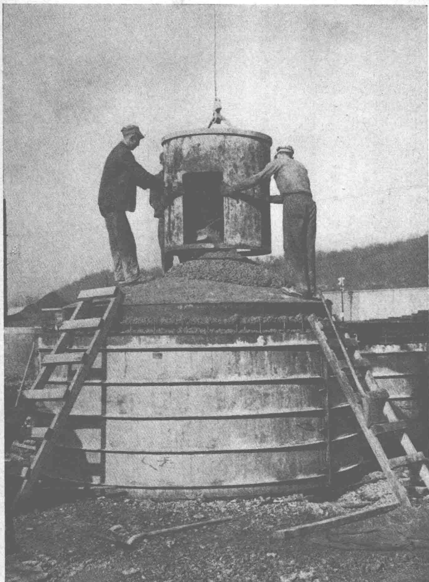
Concrete is transported from the mixer to the forms by means of a crane and bucket in this particular operation.
