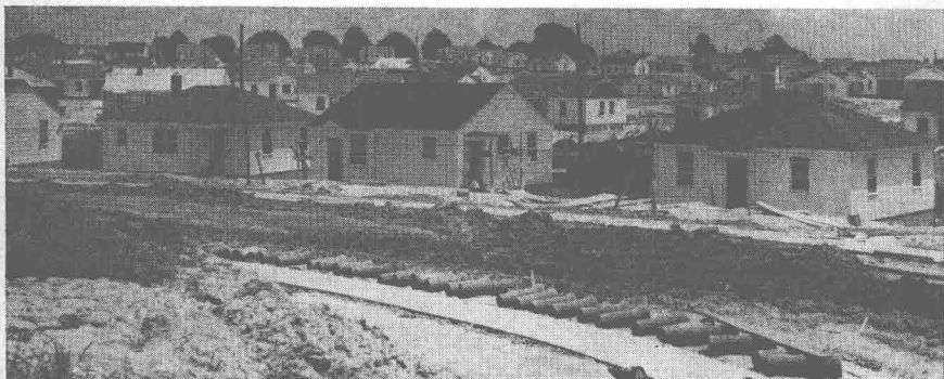
Concrete sanitary sewer pipe prior to installation on a housing development in Memphis, Tennessee.
