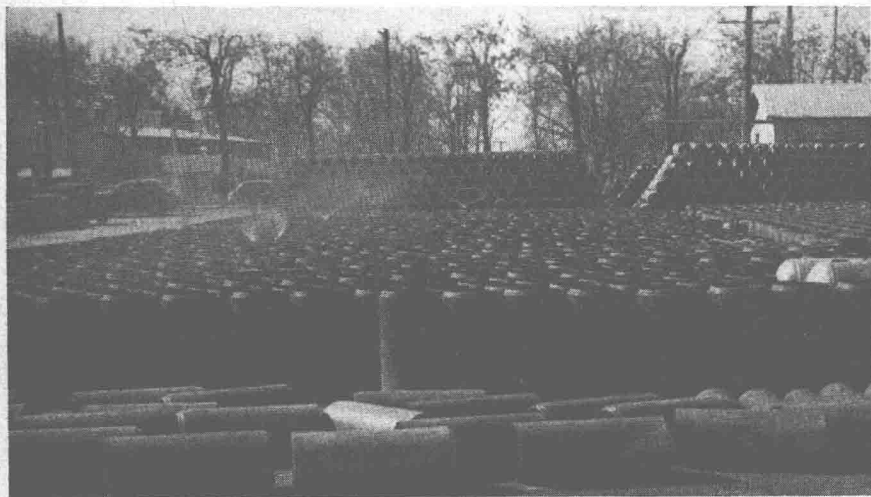
Concrete Irrigation Pipe occupies a large section of the yard above. Here sprayers are used to throw a fine spray of water over the pipe to aid in its curing.
