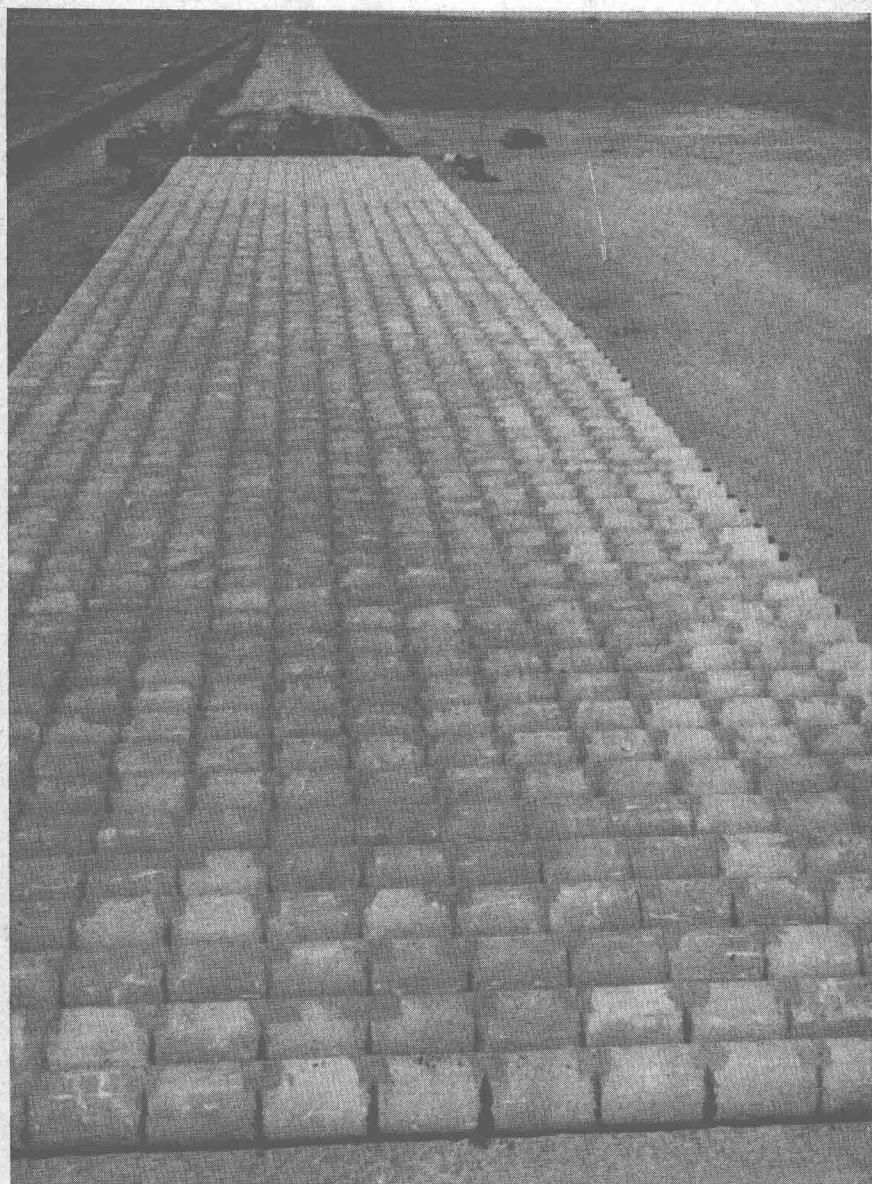
Approximately one hundred and eighty-three pipe culverts were laid on 5-foot centers to provide for drainage in the event of flash floods on an important cross-country highway in New Mexico.
